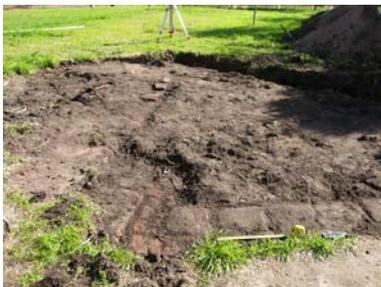
Figure 13 Brick wall footings at rear of residence (facing west).
