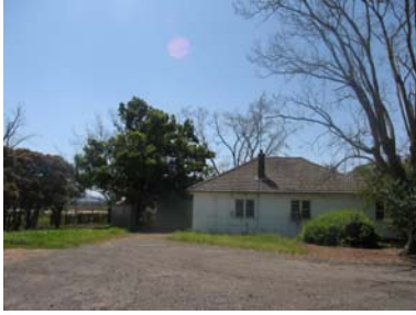
Figure 7 Fibro house north of Puddledock.
