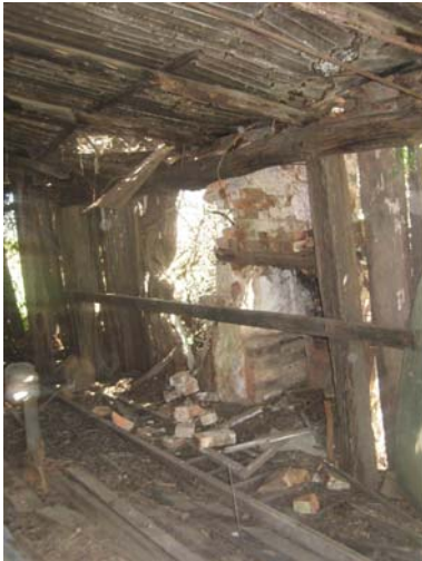
Figure 9 Rear wall of Puddledock.
