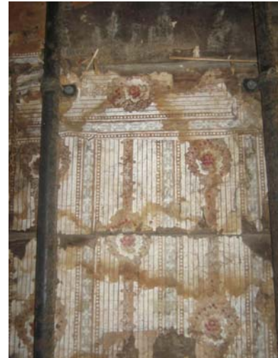
Figure 8 Wallpaper inside Puddledock.
