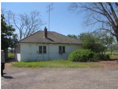
Figure 11 Fibro house north of Puddledock.
